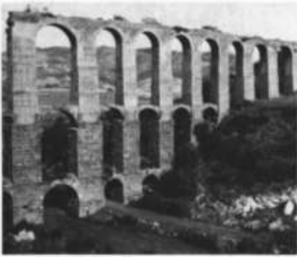
PLATE 19.3 Aqueduct from Zaghuan, which supplied Carthage
