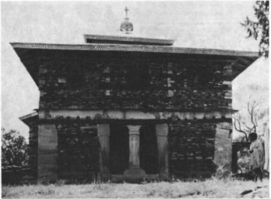
PLATE 16.6 Church of Abba Aregawi at Debre-Dāmo
